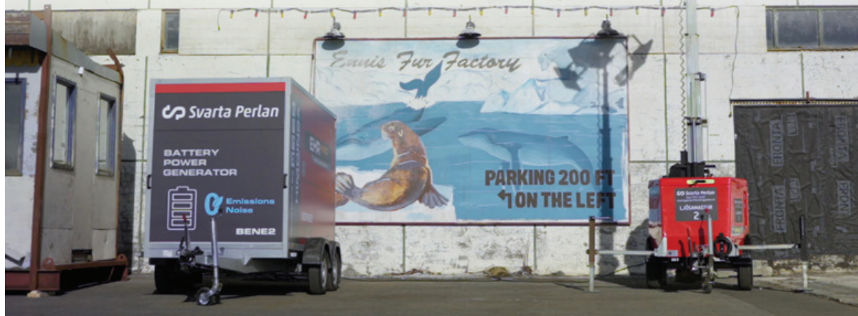
Battery-powered generators on location for True Detective: Night Country .
